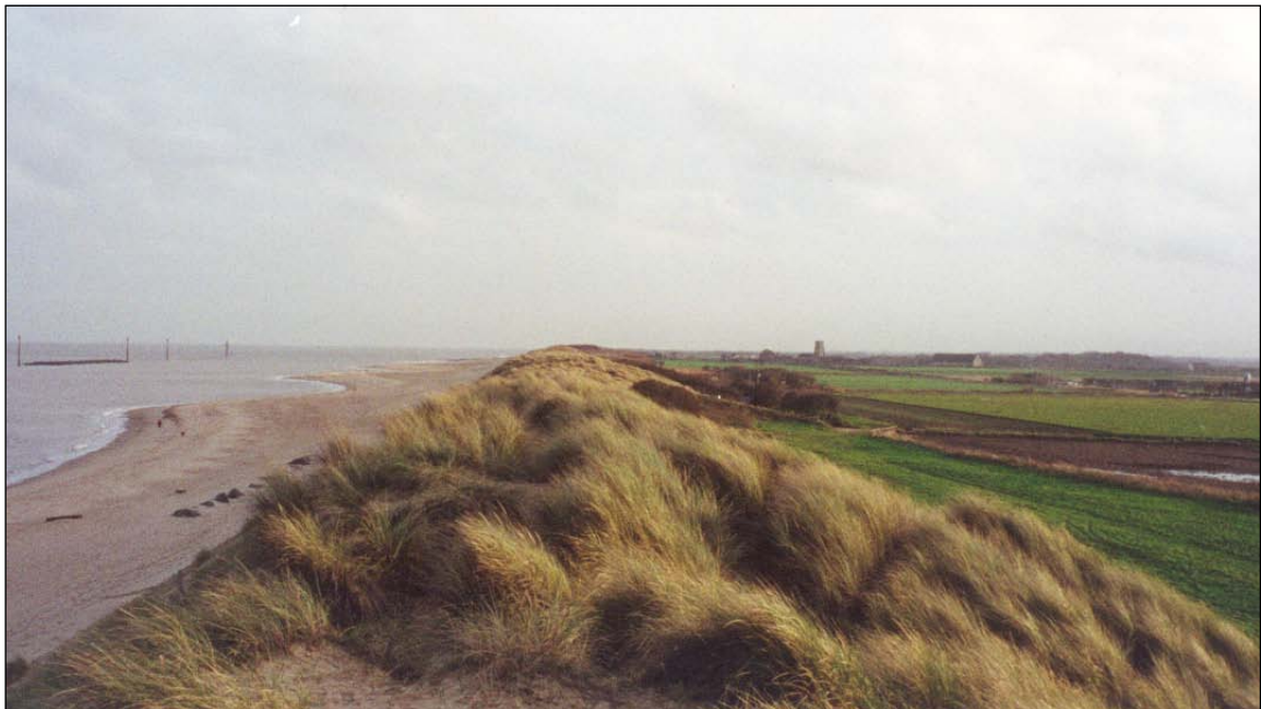
Plate 1.2 Single (partly artificial) foredune ridge, Sea Palling, Northeast Norfolk, looking south east. The dunes at this location were breached during storm surges in 1938 and 1953, resulting in loss of life and severe flooding of the agricultural land behind.
